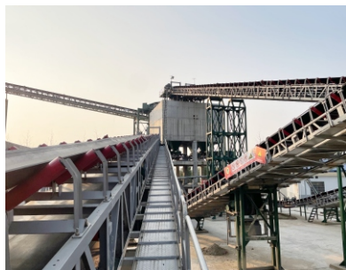
Hunan Changde Building
