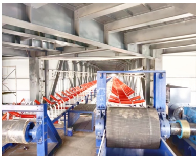
Hunan Construction Investment Hanshou Base
